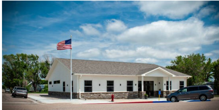
Engineering International designed a new library and city offices for Stratton. Courtesy photo
